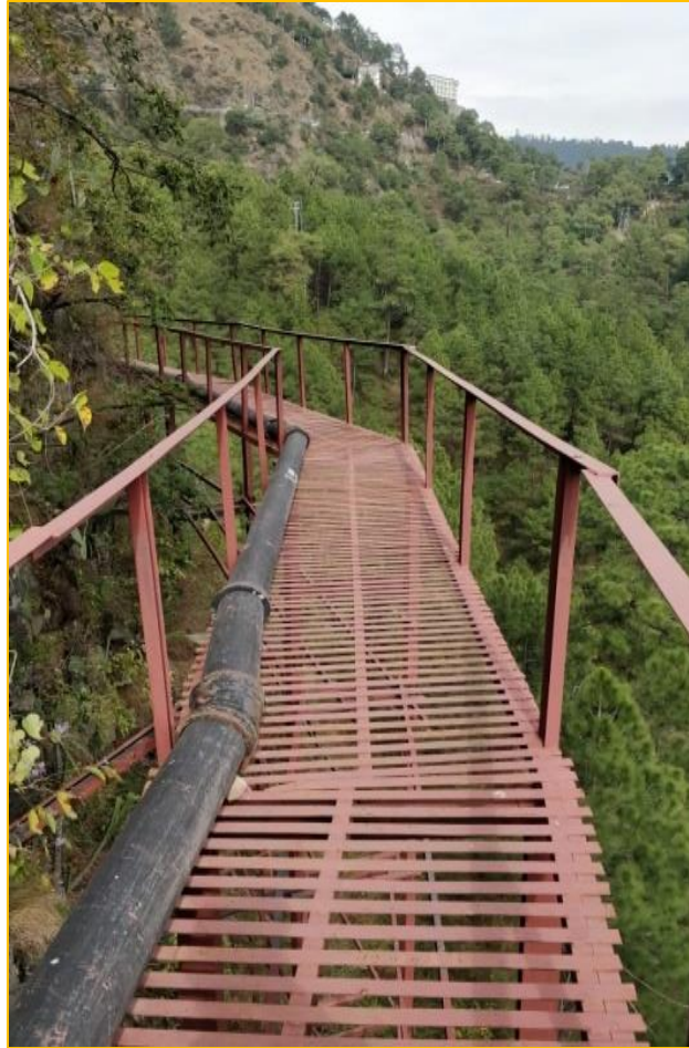
Providing and laying of sewerage DI pipes (From 100 mm to 150 mm)
