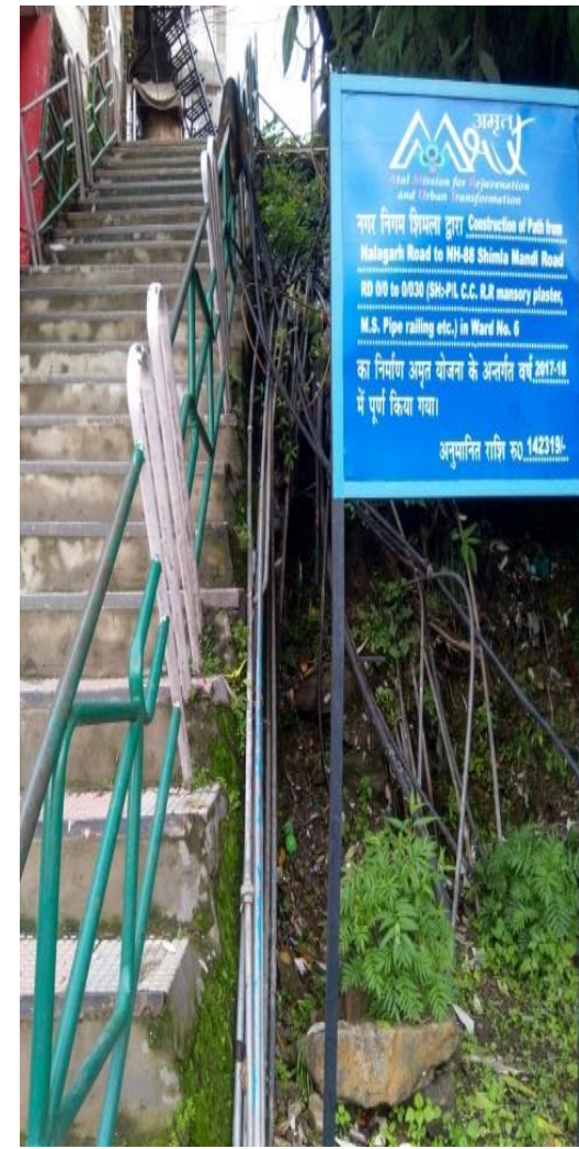
Nalagarh Road to NH 88
