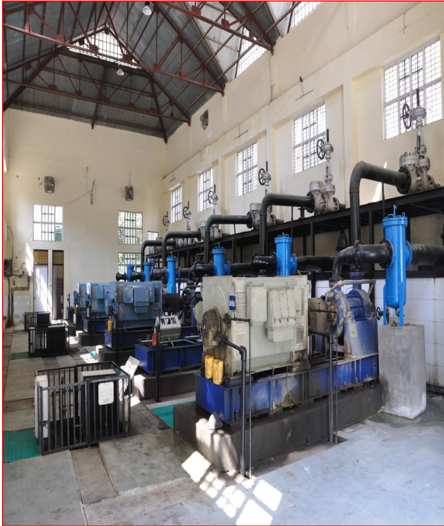
❑ 690 KW/925 HP Pumps replaced at Giri
