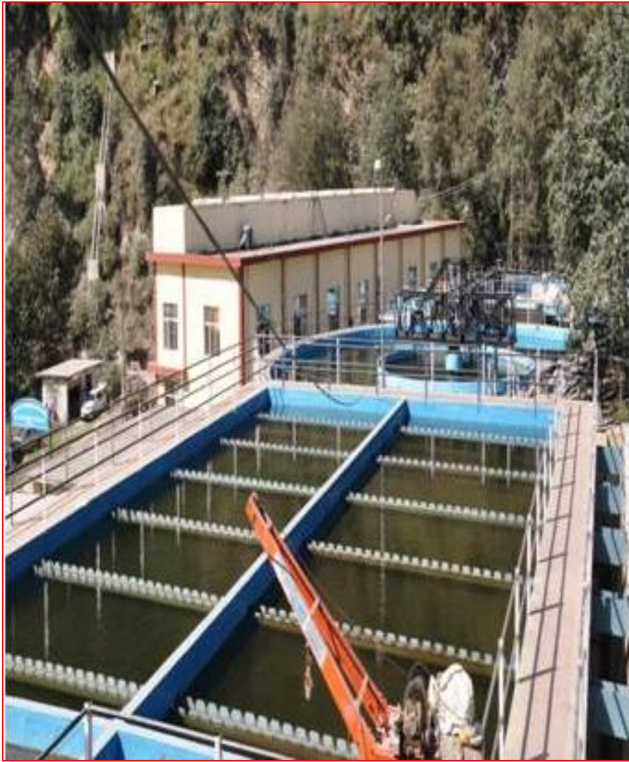
❑ Installation of Tube Settler at WTP GIRI
