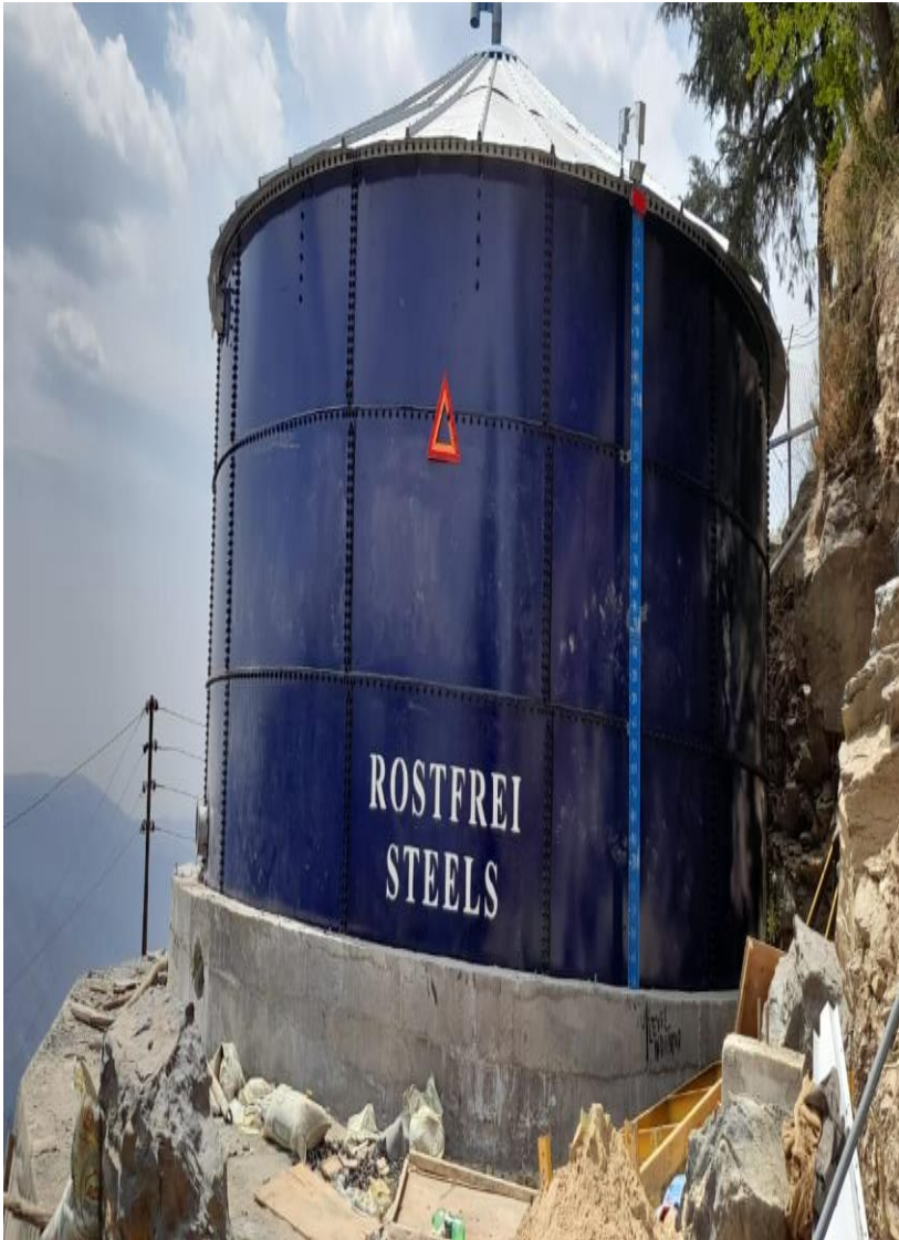
Water tank constructed at Dhingu Dhar, Sanjauli
