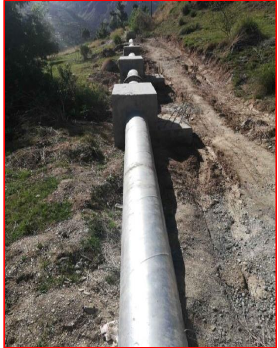
❑ 3 km rising main replaced from Majauli to Dhamandari
