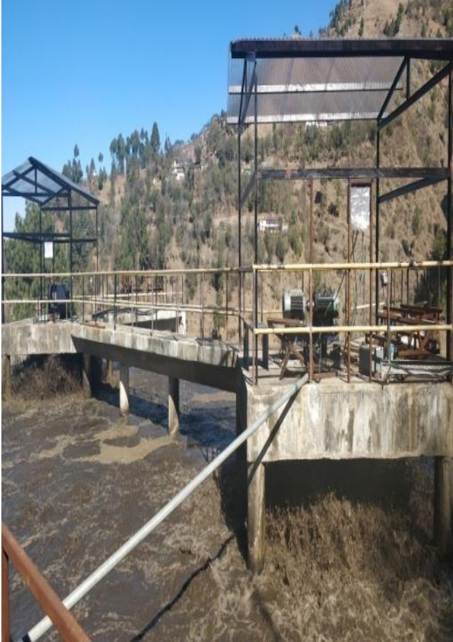
Mono submersible pump at STP North Disposal
