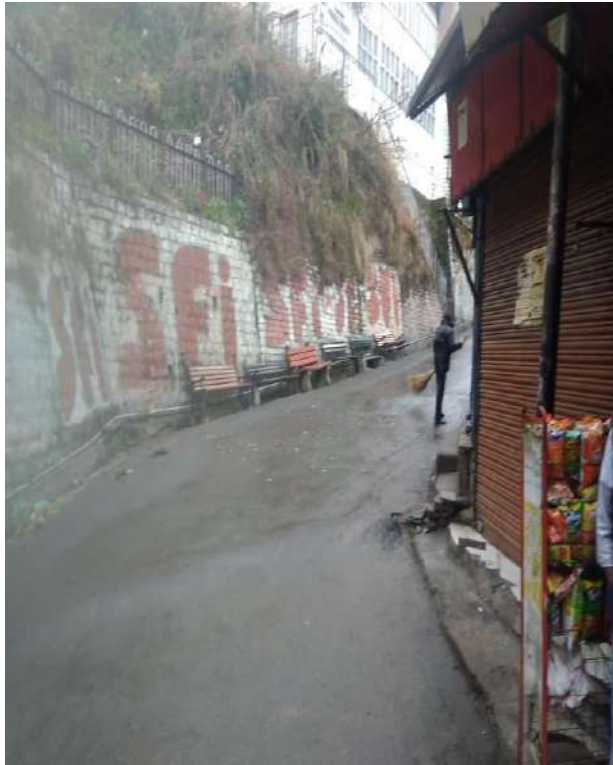
Summerhill bazar road cleaned
