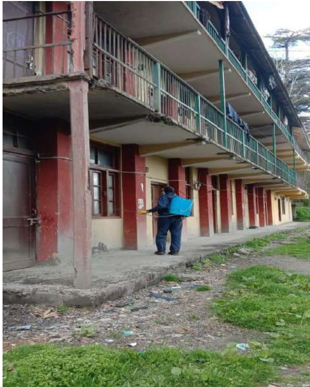
Sanitization at Labour Hostel Kothill
